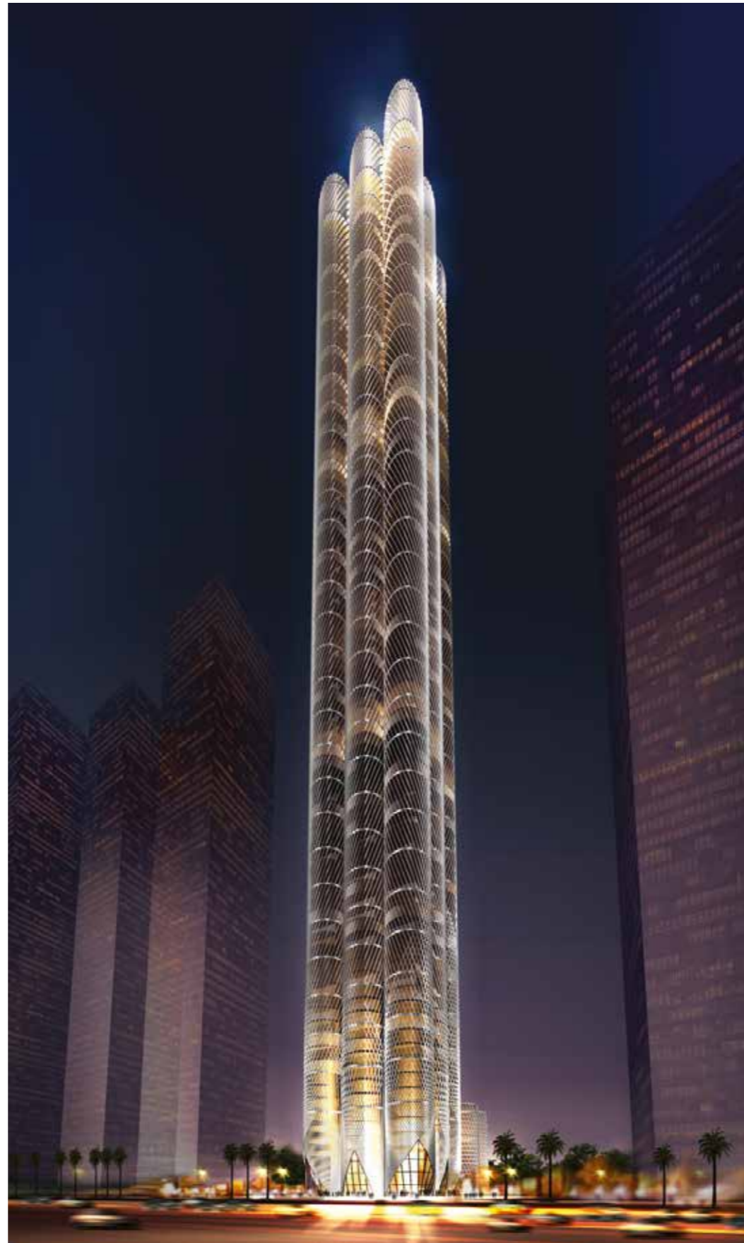
Al Sharq Tower
